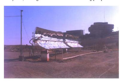
Fig.2-Typical view of the collector installed north-south direction
