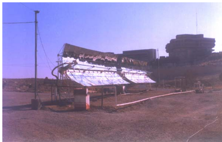
Fig.2-Typical view of the collector installed north-south direction
